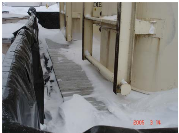
Figure 8. Fuel Storage. Fuel storage secondary containment.
